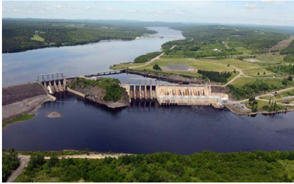
The 660 MW Mactaquac Dam in New Brunswick is in need of maintenance to extend its lifespan to 2068. PHOTO NB POWER
